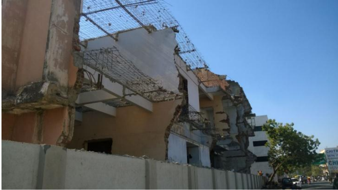
(Photo 1:- Construction and demolition site located at bhavnagar)
